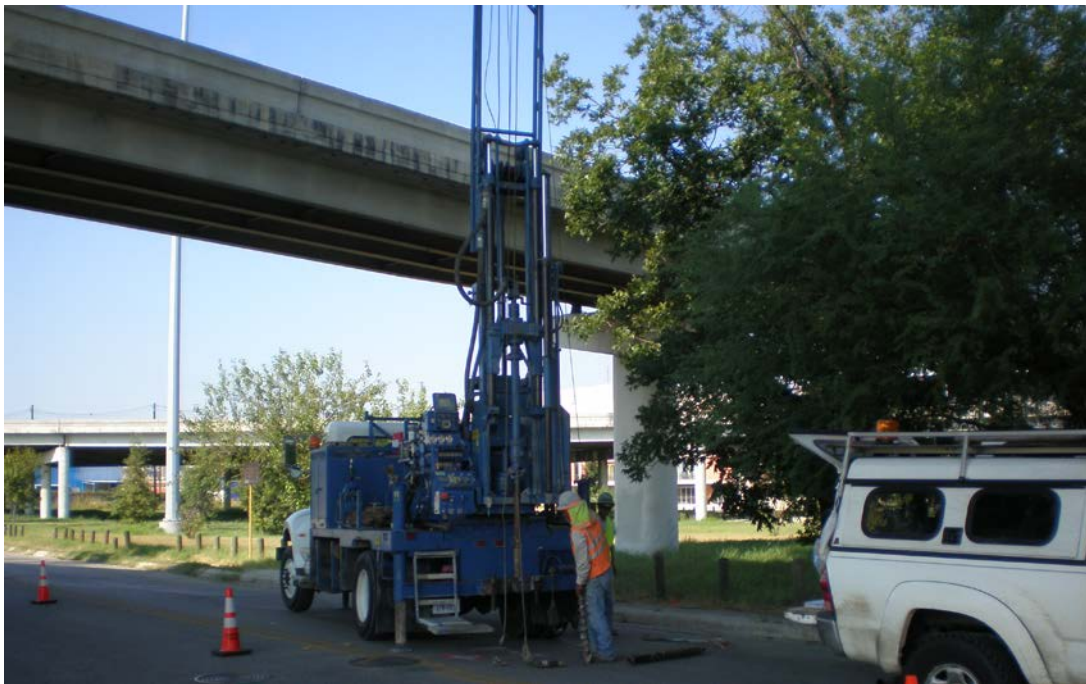
Photo 4 – View looking southwest at the drilling operations of Boring B-103.
