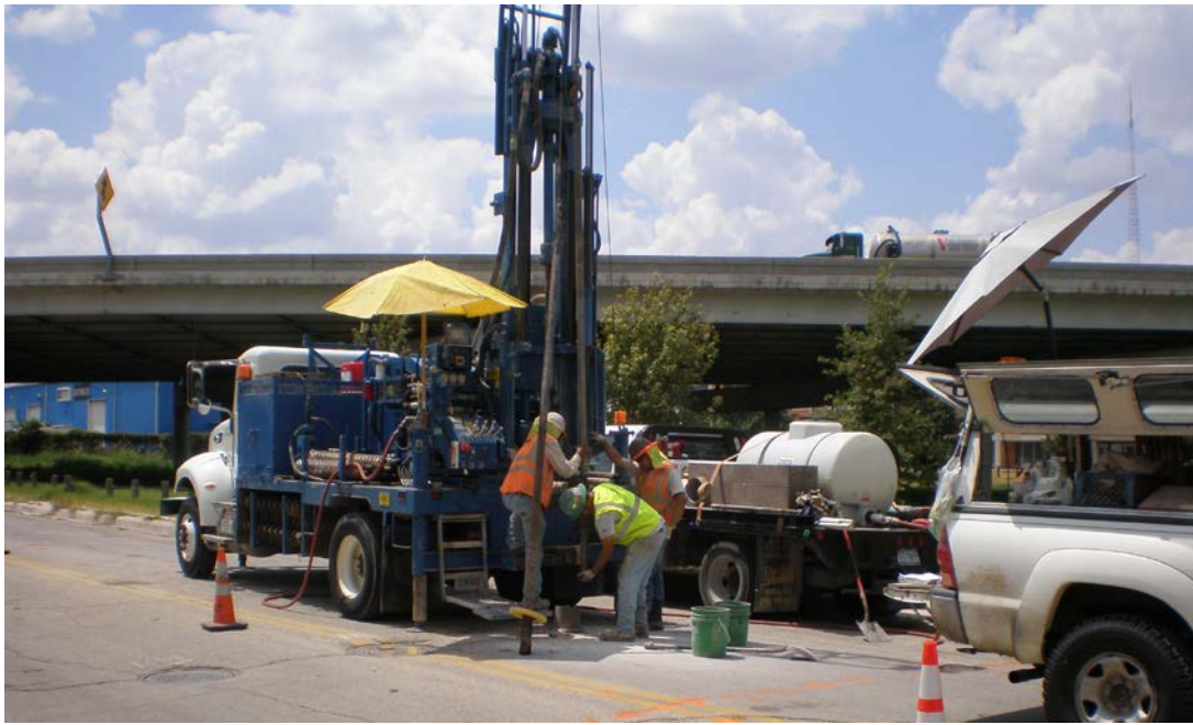
Photo 3 – View looking southwest at the drilling operations of Boring B-102.
