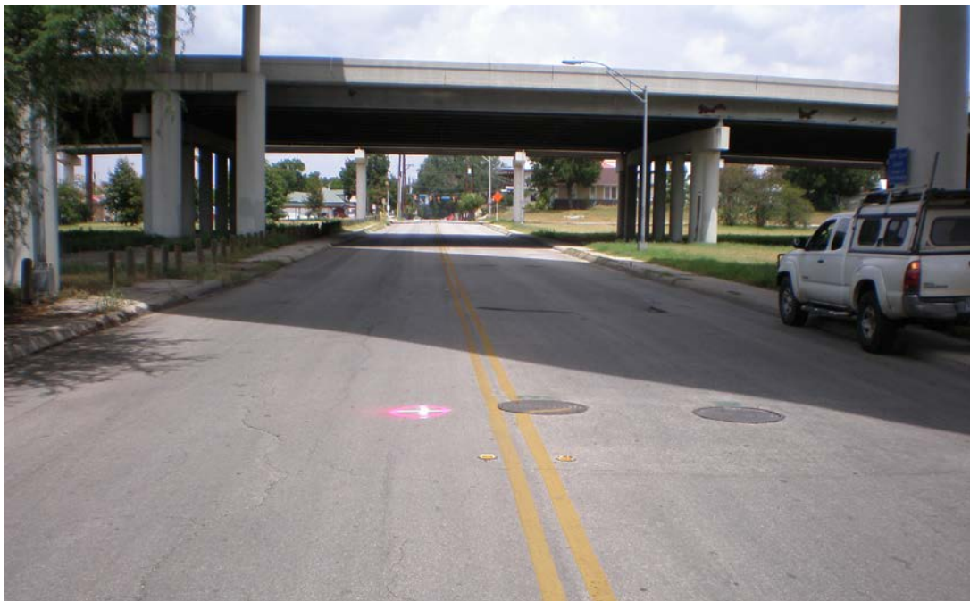
Photo 2 – View looking northeast to the proposed location of Boring B-103.
